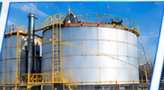
Petrochemical & Industrial Facilities
