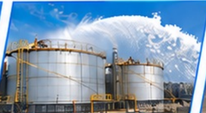
Storage Tanks & Terminals
